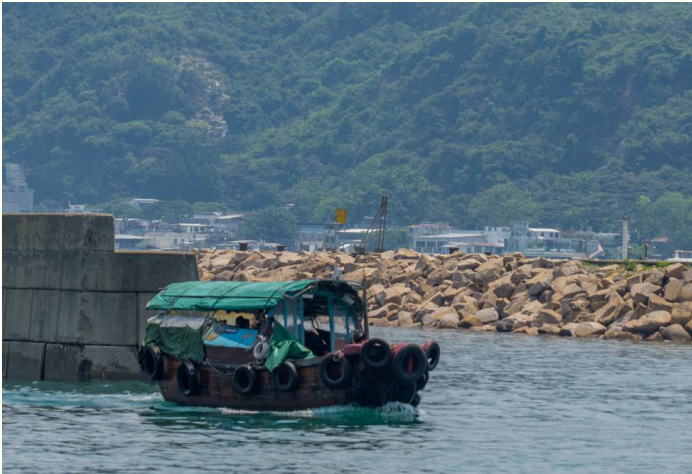
Rubble rock seawall
